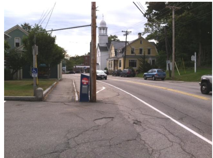
On-street Parking Restricts Sight Distance & Utility Pole Obstructs
