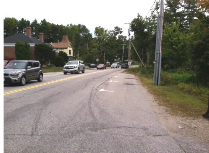
Looking North on Long Sands Road – Unprotected Utility Poles
