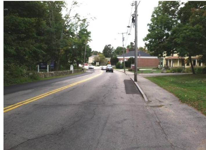
Looking South on Long Sands Road – Utility Pole Close to Travel-way
