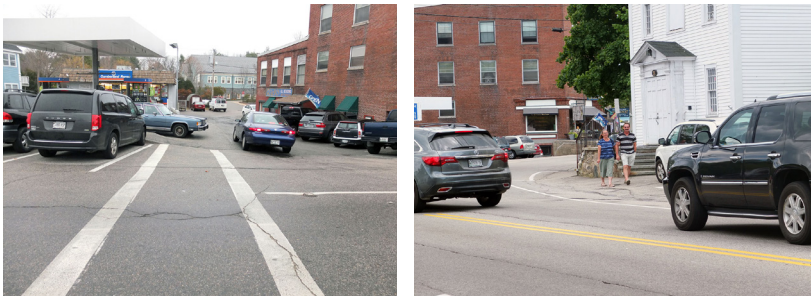
Top: Crosswalk configuration around diagonal parking. The crossing terminates at a parked vehicle; Above left: Crosswalk near Cumberland Farms; Above right: Pedestrians forced to walk against traffic.
