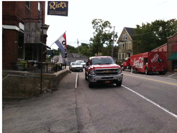
On-street Parking Restricts Sight Distance Looking Left.
