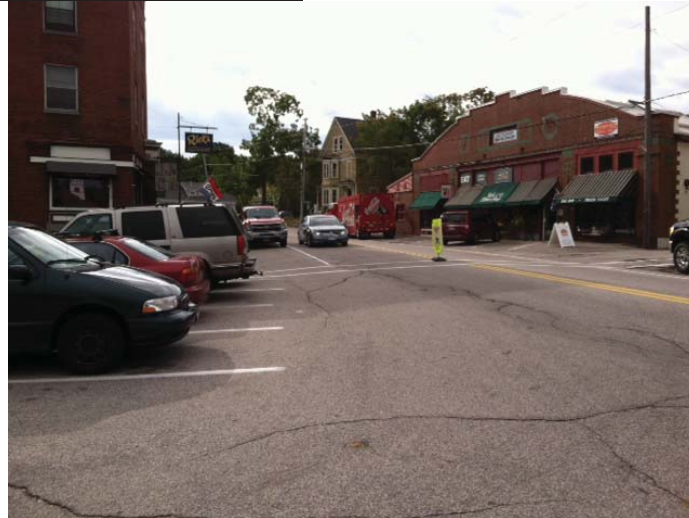
On-street Parking Restricts Sight Distance Looking Left
