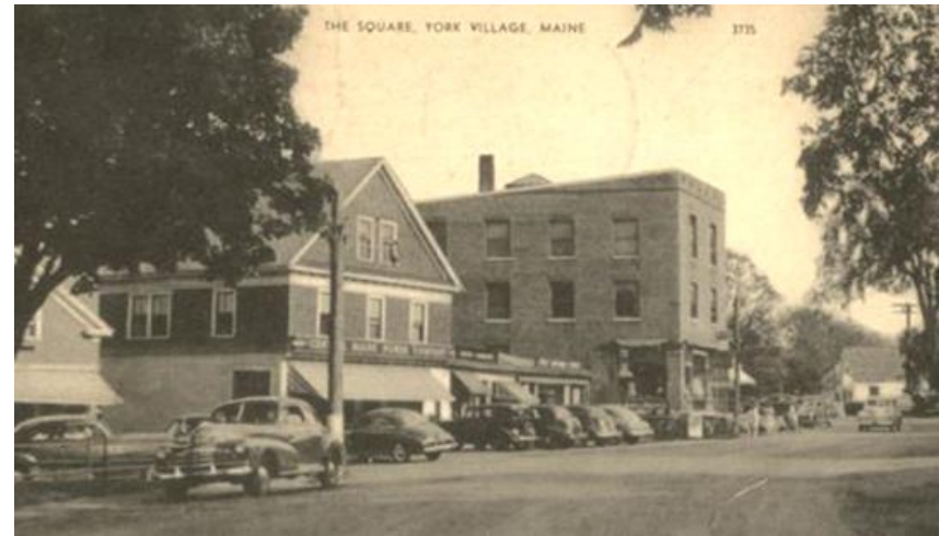
In the early to mid 20 th century, York's business district, along with the "monument square" at the intersection of York Street and Long Sands Road began to “modernize” and achieve much of its character we recognize today. Power lines and paved asphalt roads for automobiles impacted the historical nature of York Village.
