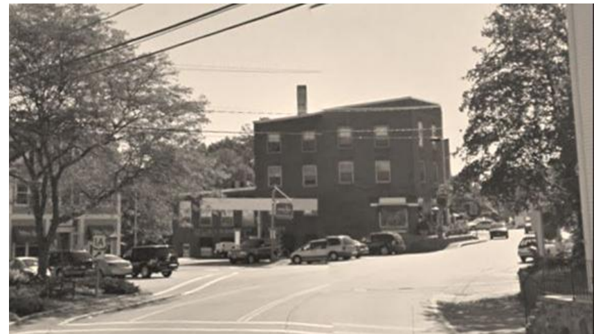
View today in the early 21 st century. Conditions have continued to evolve with the times, yet the underlying problems, and the concerns they caused, persisted. Now, almost 70 years after the 1946 Improvement Plan, its assessment of the Village as “..... inconvenient, ugly and to a degree dangerous... ” remains as appropriate as it was then.
