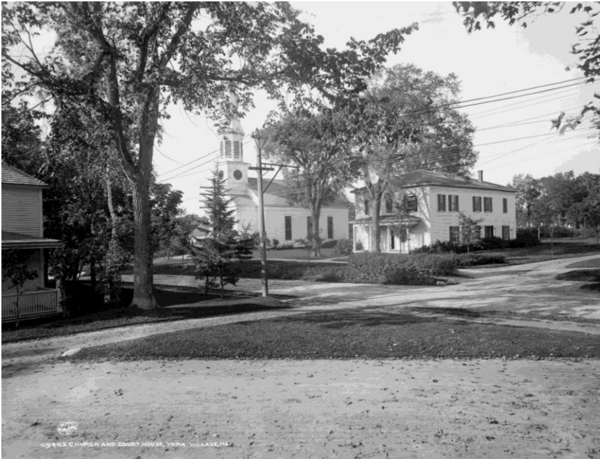
View from the intersection of York St. and Long Sands Rd, the heart of the village and future site of the Monument. Note dirt streets with electric lines. As part of a movement to beautify York, in 1882 First Parish Church was lifted from its foundation, turned perpendicular to York Street, set back twenty feet from the street, and remodeled with a new steeple.
