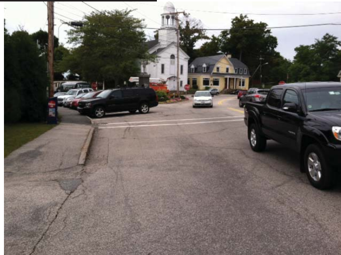
On-street Parking Restricts Sight Distance Looking Left
